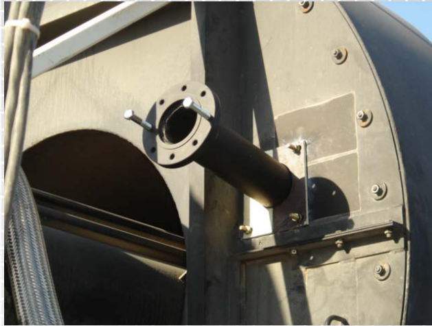
Inject Pipe Installed
