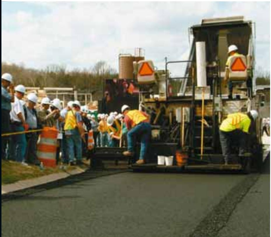
**Warm mix demonstration: At the 2004 World of Asphalt, the warm mix demonstration lowered paving temperatures approximately 80 degrees.**
